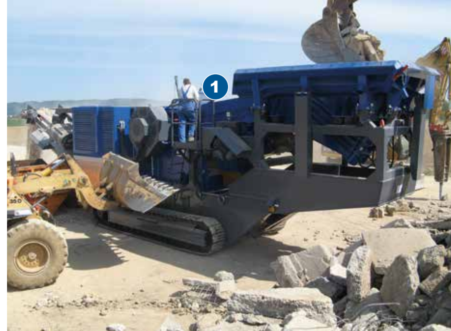
Timely intervention before material build-ups ensures smooth operation.
